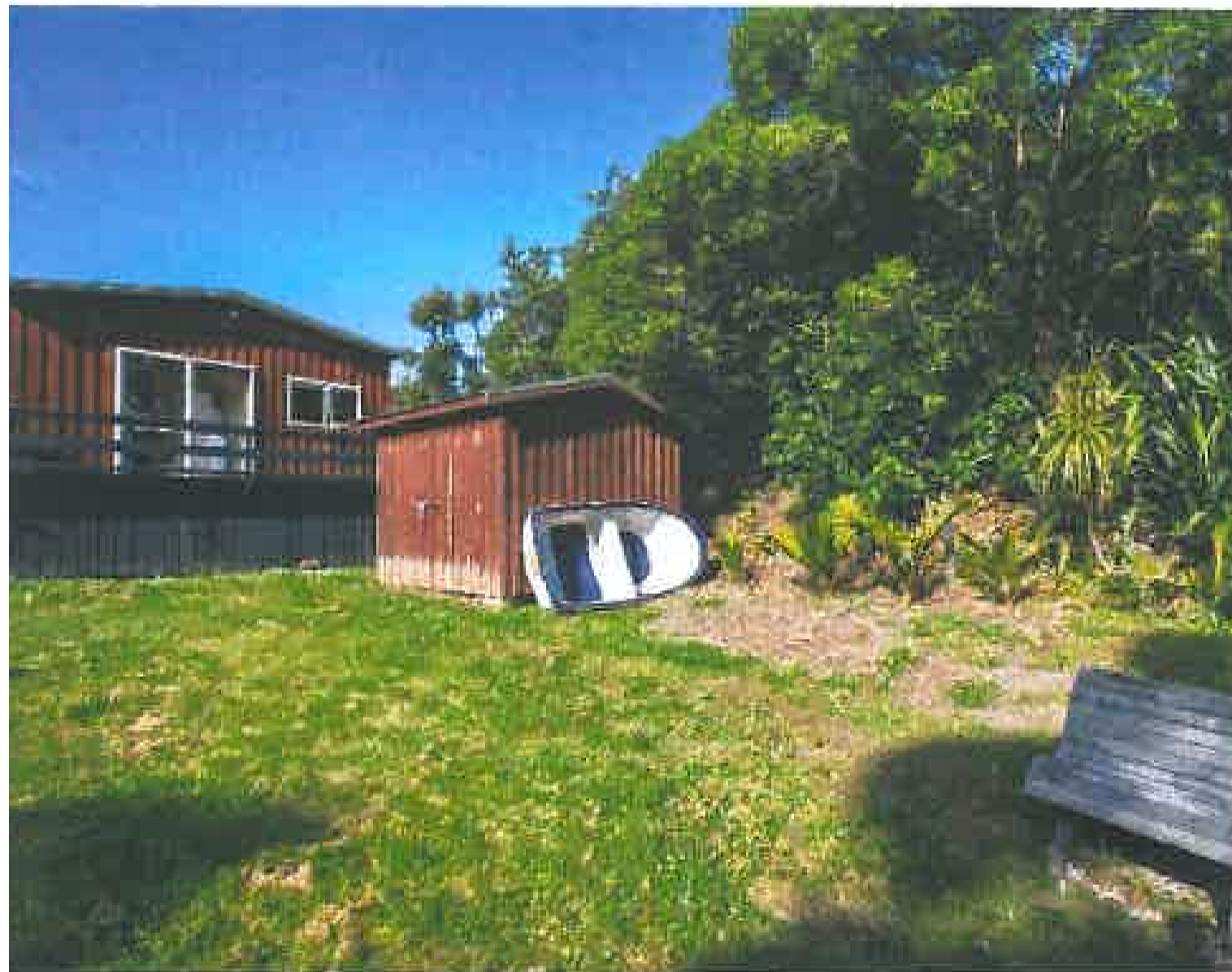
Images of existing building on site
